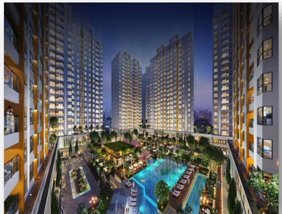
Dự án: AKARI CITY Bình Tân Nhà thầu: Công ty TNHH ĐT XD UNICONS Project: AKARI CITY Binh Tan Contractor: UNICONS Construction Investment Company Limited
